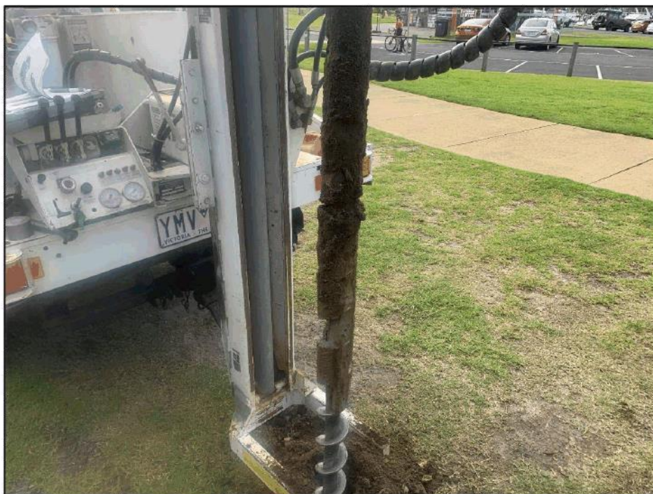
Photo 3: Drilling BH1 with the 4WD mounted Earthprobe auger drill rig
