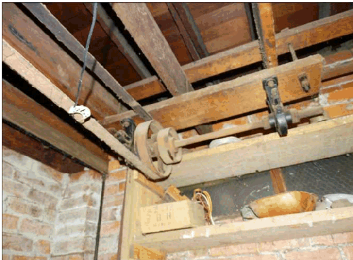
Figure 18 Line shaft attached to roof of workshop. 20
