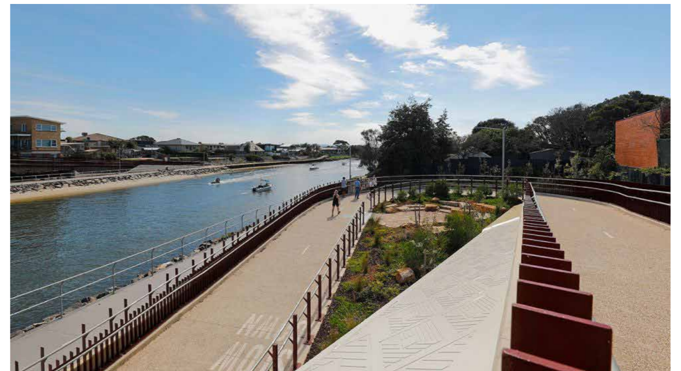
Station Street, Carrum SUP: Victoria's Big Build
