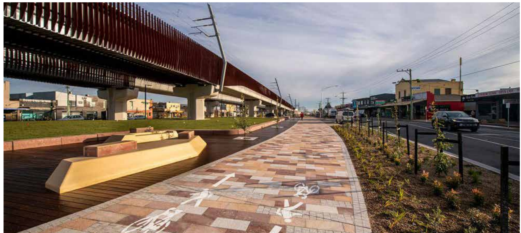
Station Street, Carrum SUP: Victoria's Big Build
