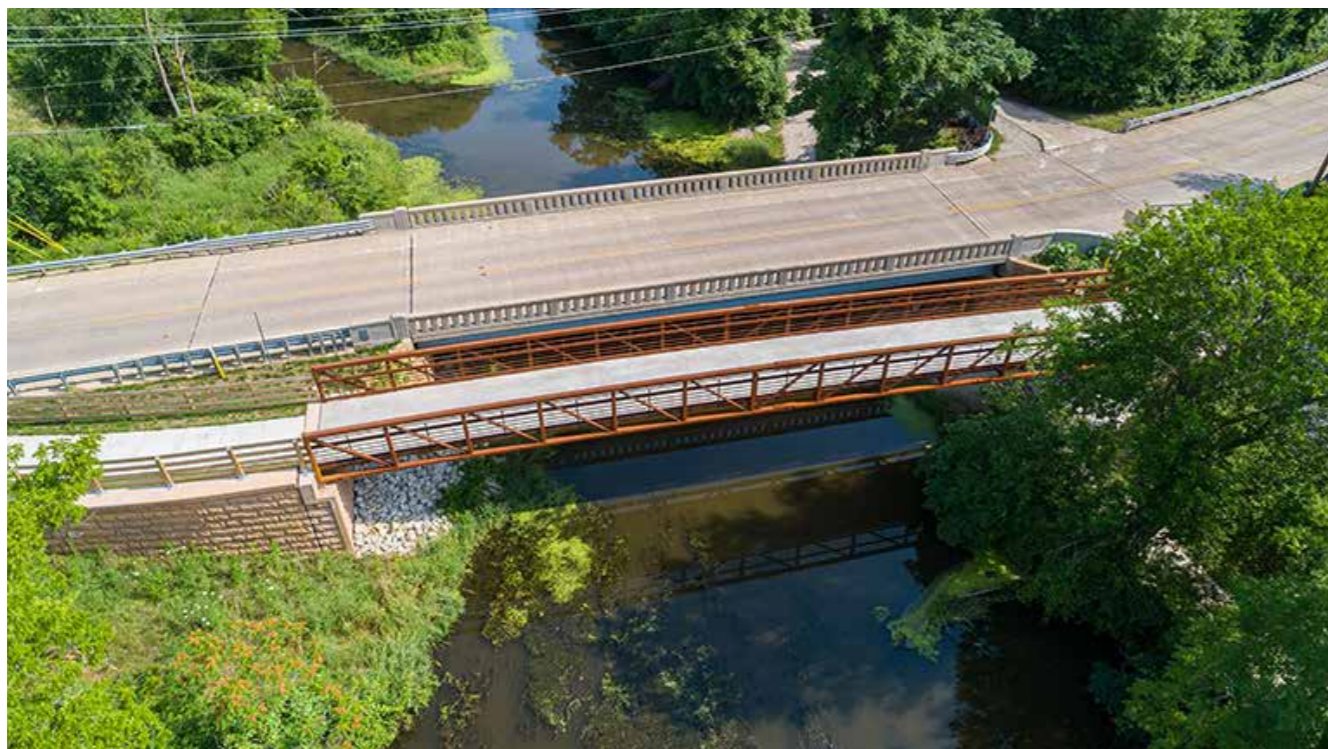
SUP bridge, Illinois US: Strand Associates
