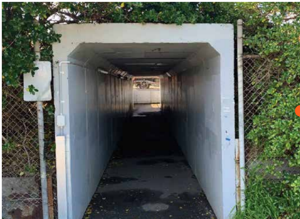
PEDESTRIAN UNDERPASS AT STABLING YARD
