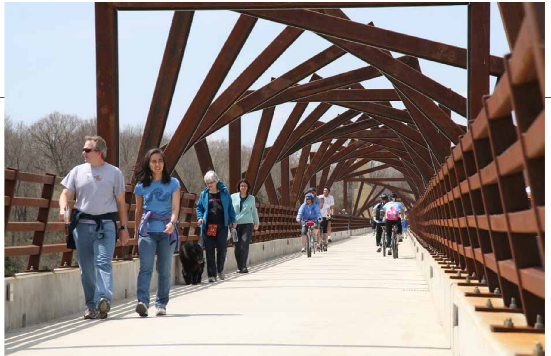
High trestle trail bridge, Prairie Trail, Iowa USA
