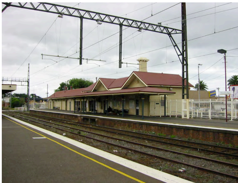
View of Upside Station Building (1882) showing double gable roof, wide verandah and long rectilinear form
