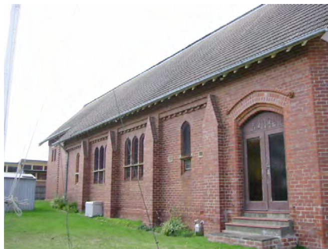
Left: East facing elevation showing arches with timber infill. Right: West facing elevation showing flat buttresses, lancet arched windows and label mould above door.
