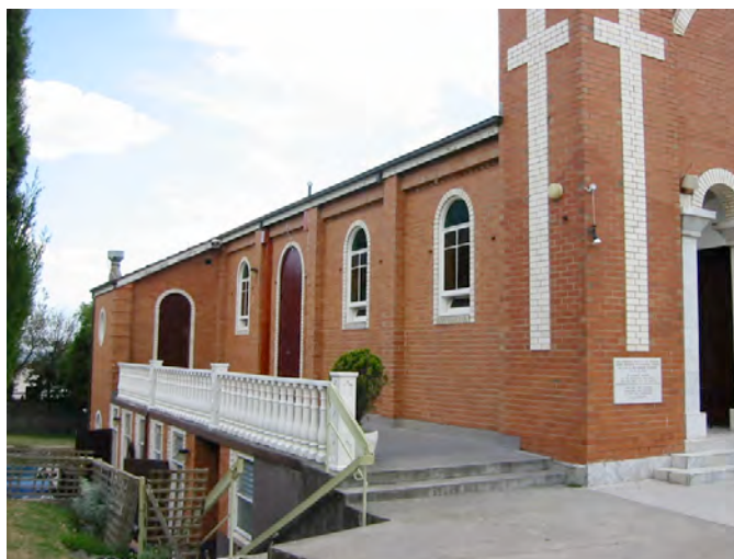
Side view of church showing simple arched windows and doors with white brick trims.
