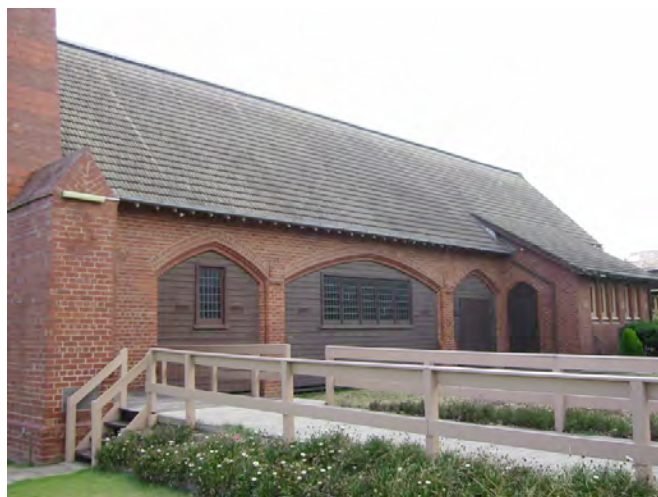
Left: East facing elevation showing arches with timber infill. Right: West facing elevation showing flat buttresses, lancet arched windows and label mould above door.
