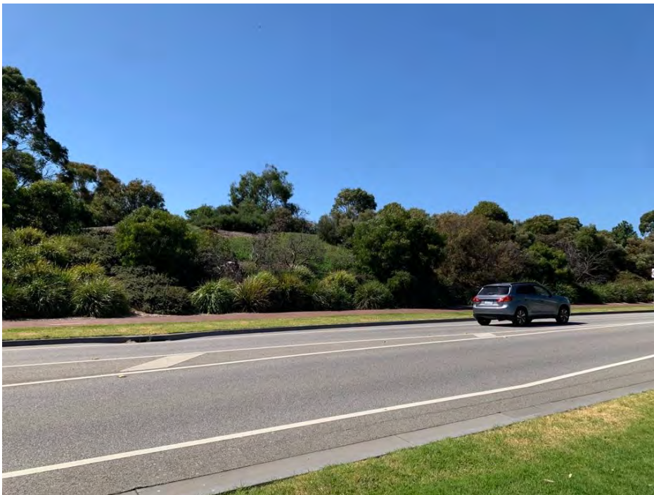
Existing raised vegetated buffer on the north side of Governor Road
