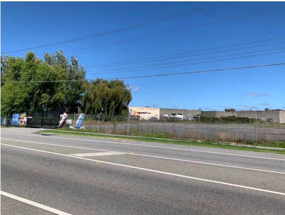
Subject site (1-7 Wells Road) from Governor Road (photo by Planning Officer)
