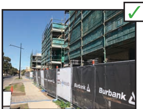
(c) Shade cloth is on scaffold. 1. Fence & feet are behind property line.
