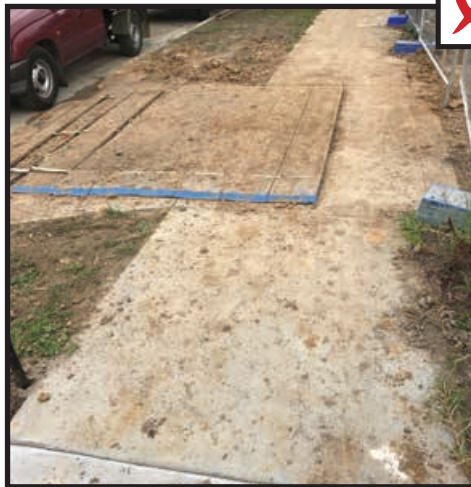
Example of dirty footpath and crossover protection which needs cleaning and repairing
