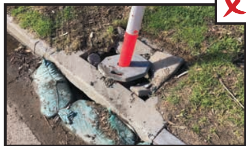
Damage to Council Side Entry Pit.
