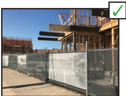
(c) Shade cloth is appropriately fixed to fence.
