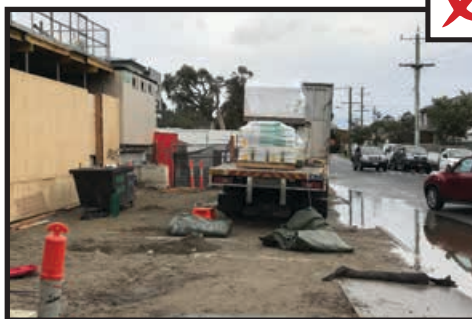
Builders have: caused flooding and blocked Council drainage system, removed footpath, occupied Council land without a permit, have unsecured items lying around the site and have not kept footpath hazard free for pedestrians.
