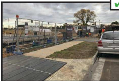
Example of timber crossover protection in good condition.
