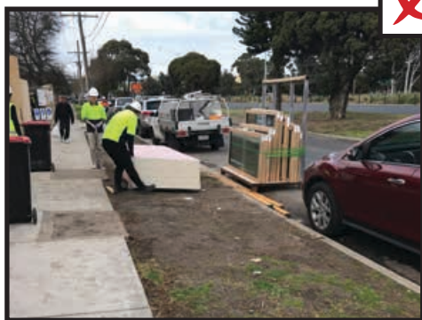
Building materials should be unloaded from within the site and should not be left on the naturestrip or road unless a permit has been obtained.
