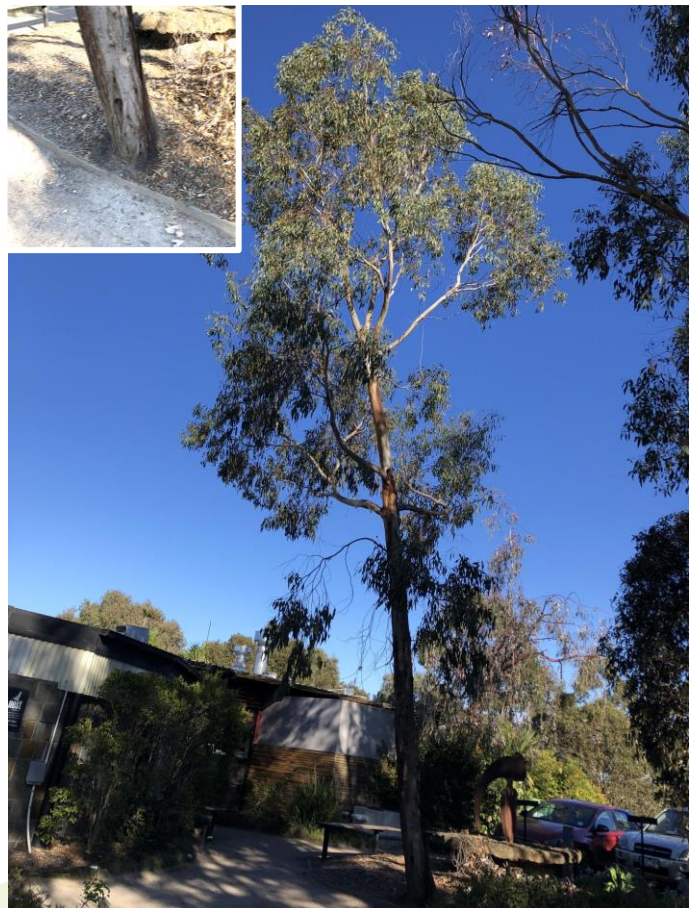
Image 13: Tree 666, poorly located Swamp Gum in one of the highest use areas in the estate near café; tree has insufficient space (see inset). Recommended for removal within 12 months.
