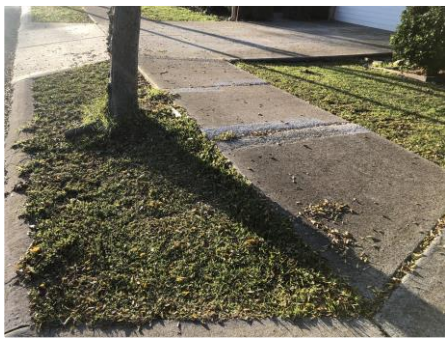
Image 6: Tree 325, Chinese Elm south of Arcots Court planted far too close to kerb despite ample space further away, increasing likelihood of root damage and also blocking access for car users. Tree recommended for removal.
