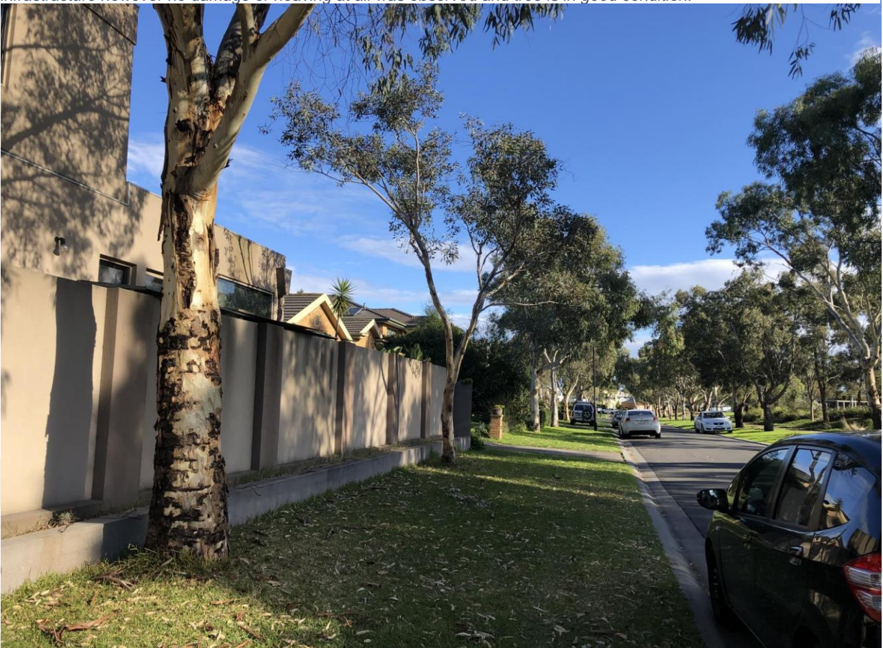
Image 9: Trees 1999-2000, River Red Gums along Lake King Circuit planted adjacent to property boundary and as a result being far too close to boundary walls of this property. Trees recommended for removal.
