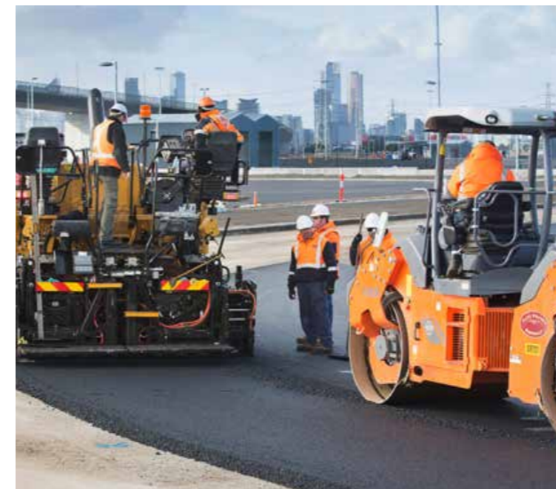
Recycled plastics and glass are used in this new road-base (via Sustainability Victoria).
