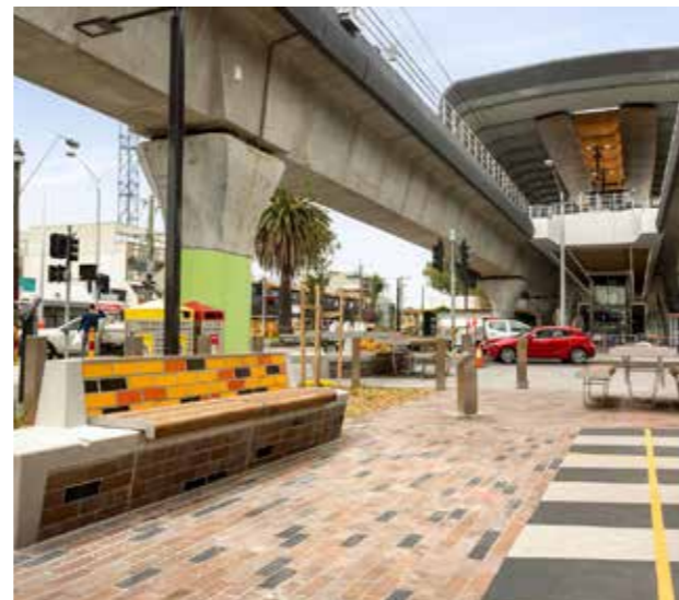
Clayton Station along the completed Caulfield to Dandenong LXR.
