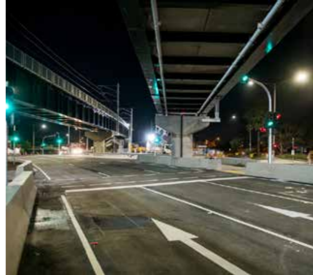
Steel girders at Reservoir LXP help to reduce visual bulk of viaducts.
