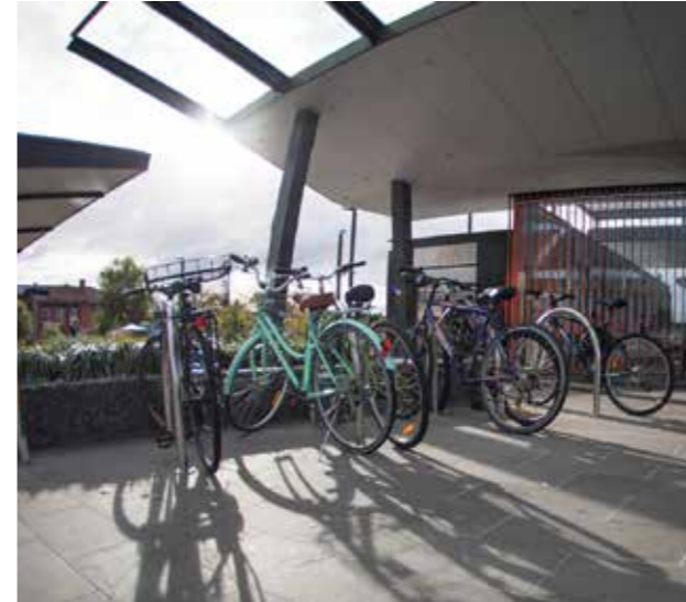
Singular bicycle parking loops at Ormond Station with adequate spacing. An undercroft location is ideal.
