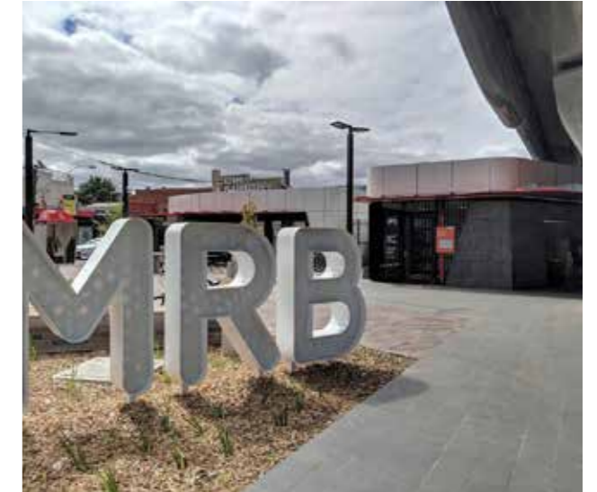
The signage at Murumbeena Station and others as part of the Caulfield to Dandenong LXP is a feature.
