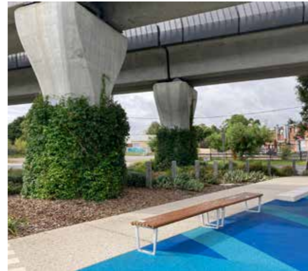
Vertical greening of elevated rail columns.
