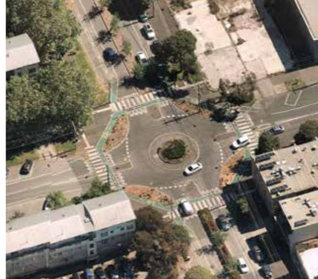
Improvements to roundabouts at Cecil Street, South Melbourne, allow safe crossing opportunities for people walking and cycling while providing legibility for motorists navigating the area.
