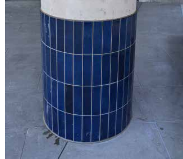
The tiles on this concrete column create a more fine-grain finish that is sympathetic to a village character.
