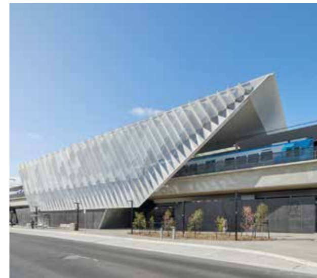
The completed Reservoir LXR.
