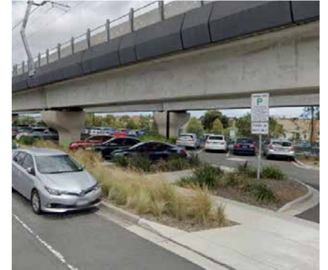
Accessible parking at Clayton Station.
