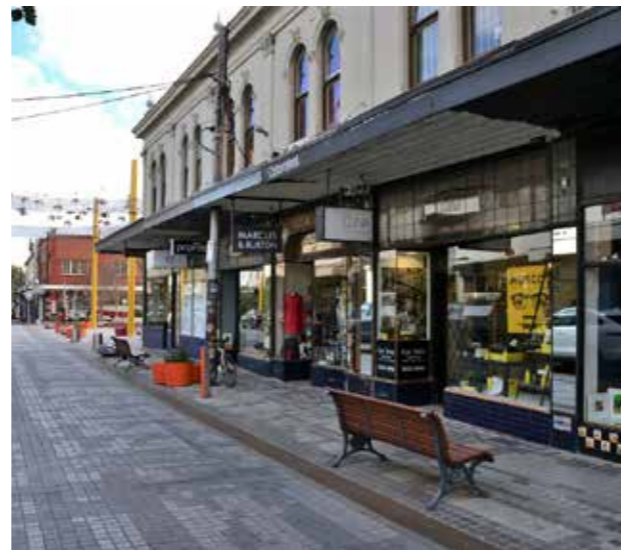
New streetscape works that complement adjoining heritage buildings and prioritise pedestrians.
