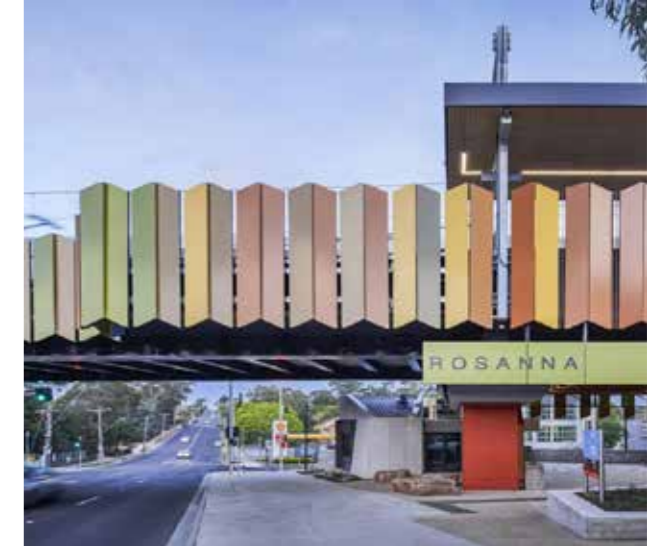
Vertical articulation at Rosanna Station helps to break down the volume of the station.
