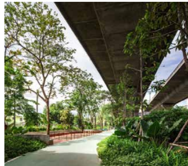
Shared user path bordered by generous planting beneath elevated motorway.
