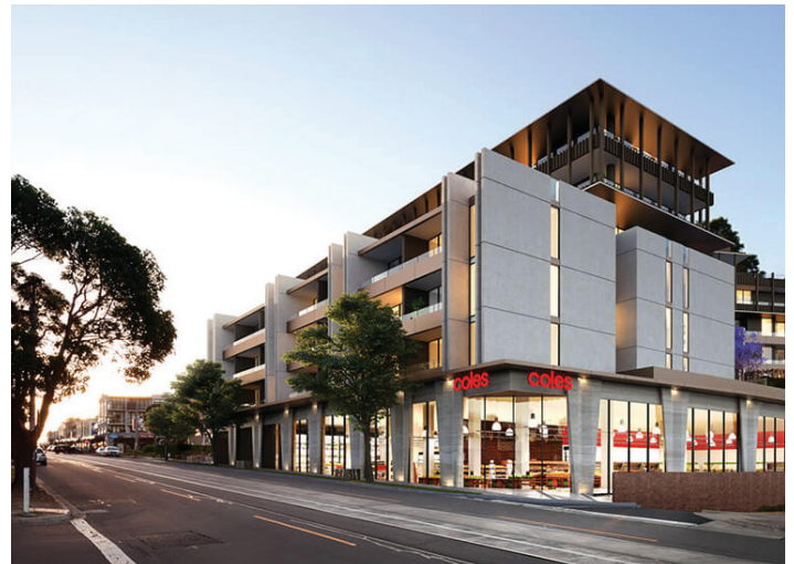
Examples of mixed use development in a podium- tower format, with supermarket at ground level in Kew (by Fender Katsalidis Architects)
