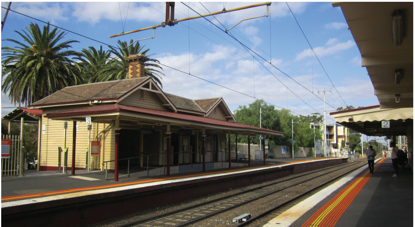
Existing heritage station building (east siding)
