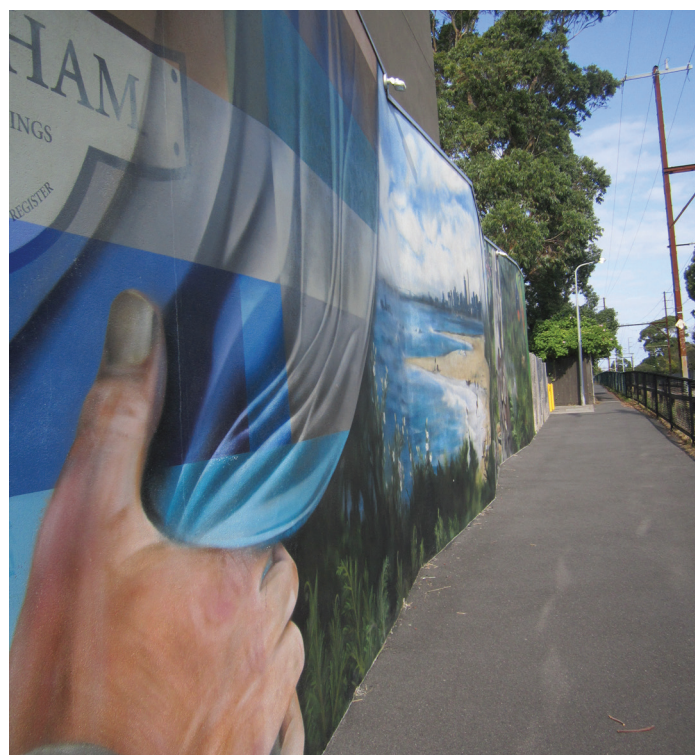
Existing pedestrian footpath along railway line
