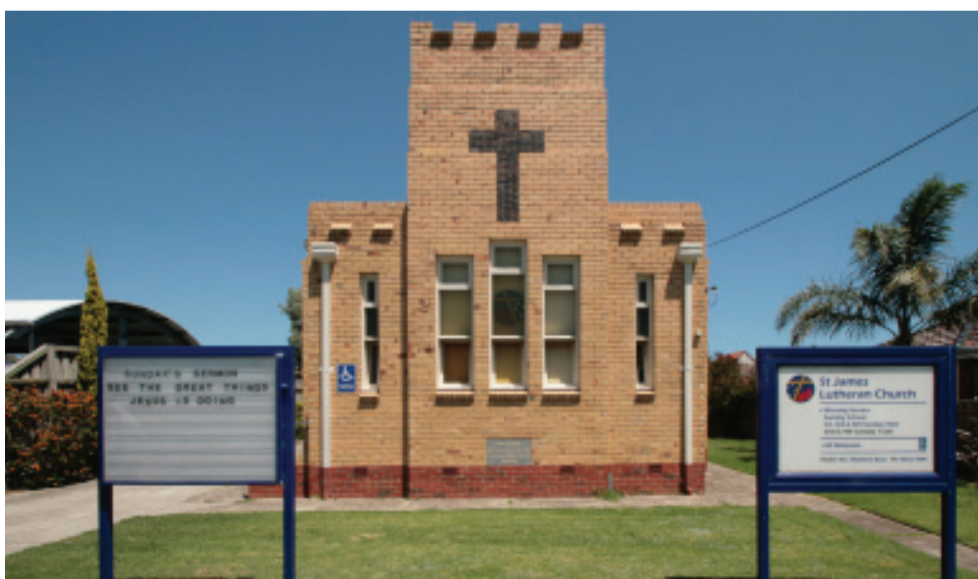
Heritage listed St James Lutheran Church, located immediately adjacent to the South Road boundary (protected by a heritage overlay HO 118)
