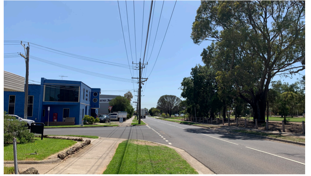
View along Linton Street, looking north. The large format warehouse retail presents an inactive frontage to the street.
