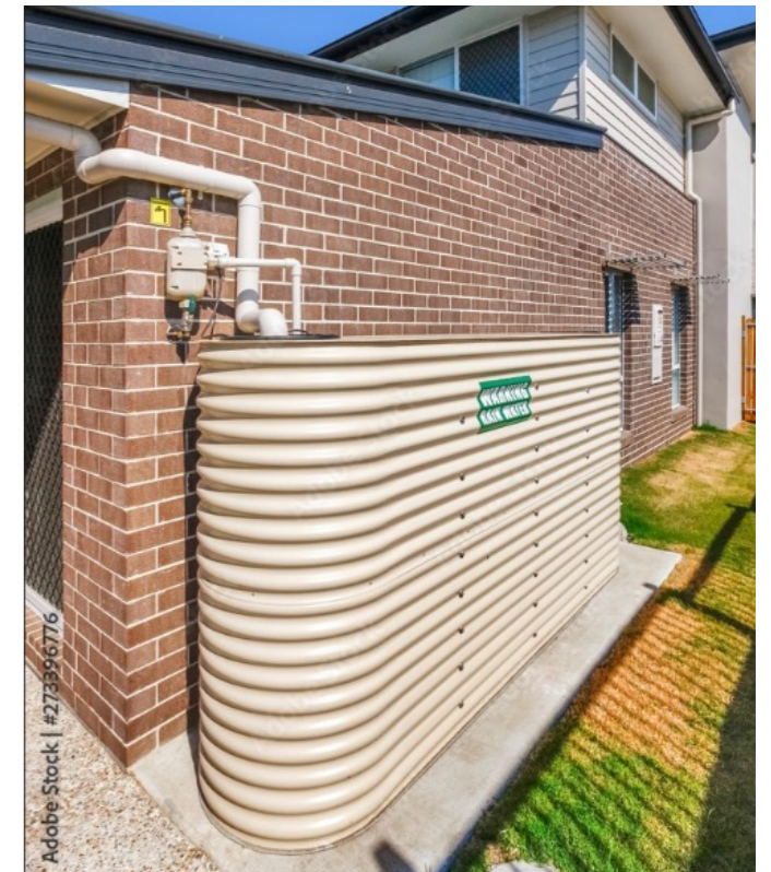
Figure 7. Slim rainwater tank
