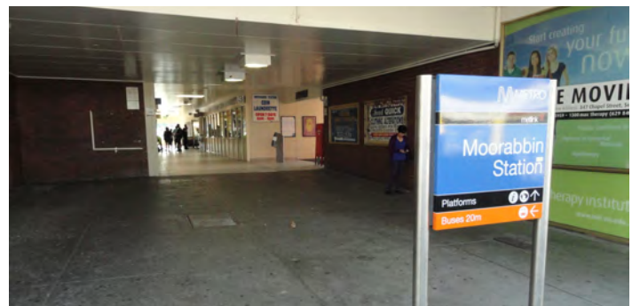
Typical signage and dark undercroft spaces to station entry
