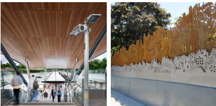
Example of shelters and fencing within a station precinct
