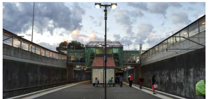
Blank concrete walls along platform and glazed concourse above
