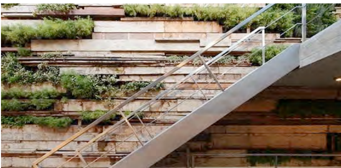
Example of finishes to trench walls at platform level
