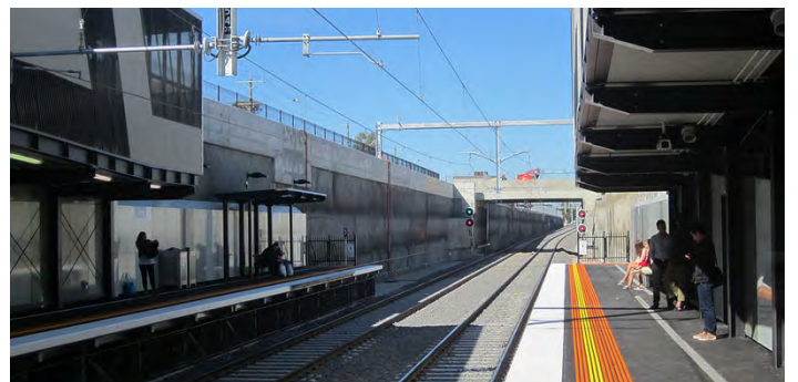
Blank precast concrete walls along platform
