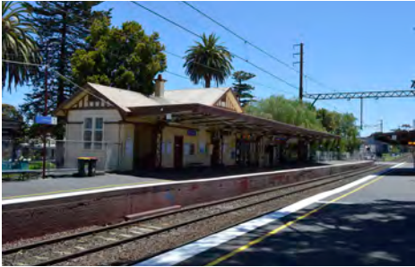
Platform 1 and heritage station building
