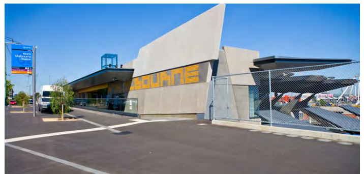
High precast concrete walls inconsistent with preferred Mentone character
