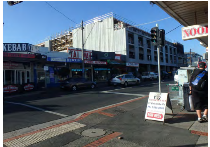
Figure 17. 4 storey mixed use building under construction on Balcombe Road
