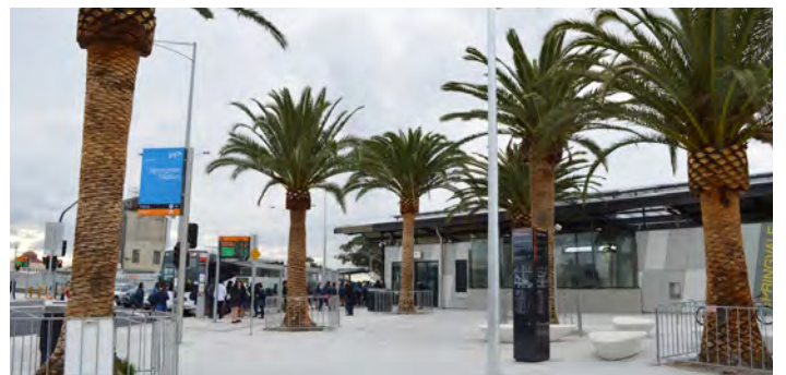
Station forecourt comprising impermeable surfaces with minimal visual interest
