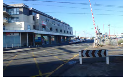
Level crossing condition to Balcombe Road
