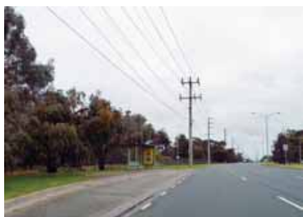
FIGURE 18 EXISTING BUS SOPS WITHIN THE GREEN WEDGE
