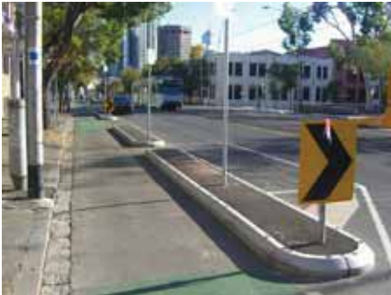
FIGURE 19 EXISTING BUS SOPS WITHIN THE GREEN WEDGE
