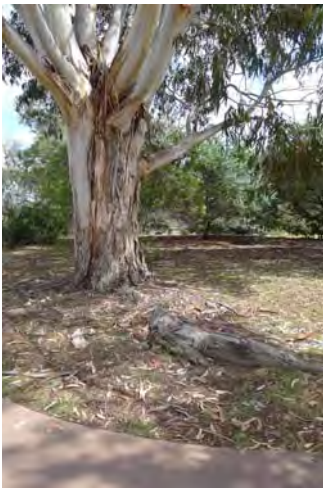
Photo 79 from east: Tree 86 large surface root
