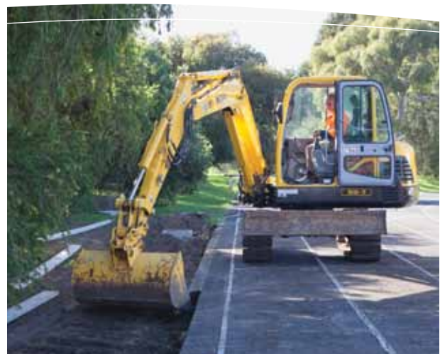
As part of Kingston's Capital Works program, Bricker Reserve athletics track in Moorabbin underwent an upgrade at a total cost of $271,000.
