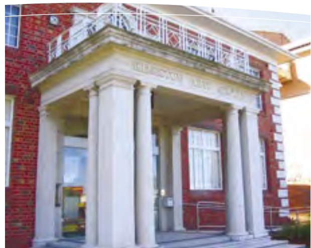
Kingston Arts Centre on the corner of South Road and Nepean Highway, Moorabbin was once the location of the former City of Moorabbin Council Chamber.
