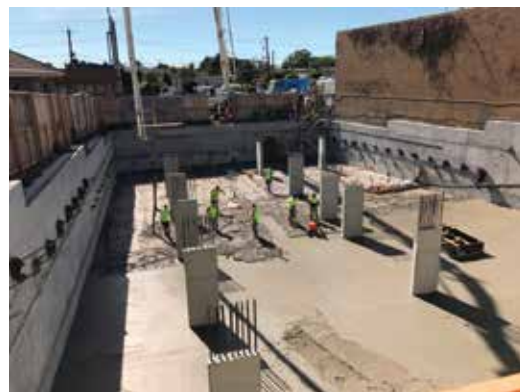
Basement Concreting works at a development in Main St, Mordialloc
