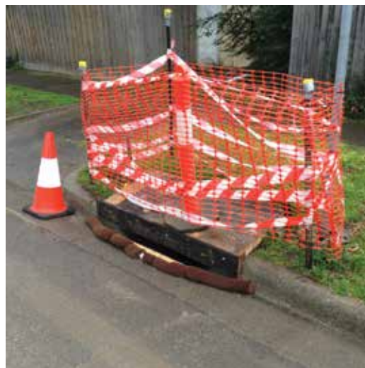
Protection of Council drainage pit in Cheltenham
