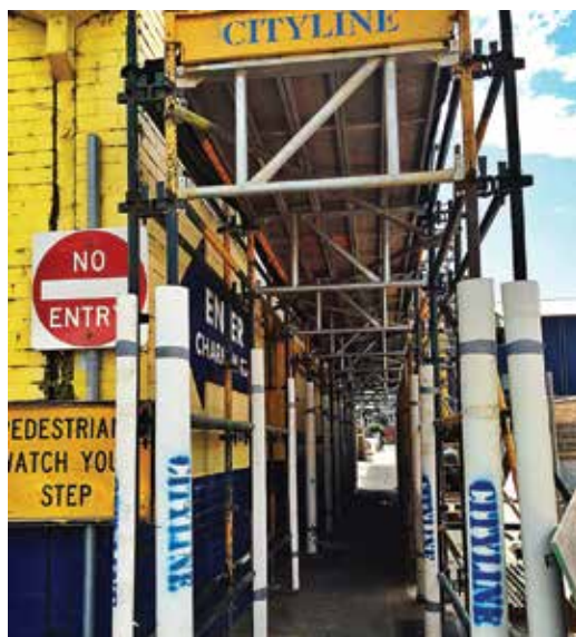
Example of overhead scaffolding for Cheltenham Development
