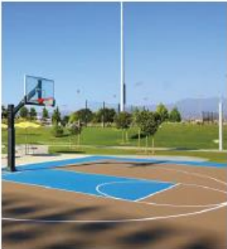
Coloured surface and linemarkings to basketball court
