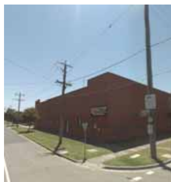
Rear of the Mentone Tenpin Bowls building from Childers Street
