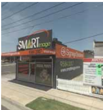
Commercial building that adjoins the Subject Site to its east
