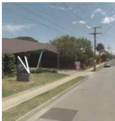
Vet Clinic located on the south side of Balcombe Road
