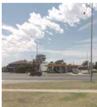
Mentone Fire Station & Shell Service Station on the eastern side of the Nepean Highway
