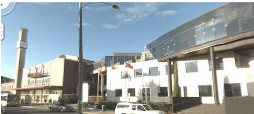
Refurnished Commercial Building at No. 999 Nepean Highway, Moorabbin
